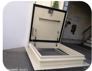
Roof access Hatch cover
